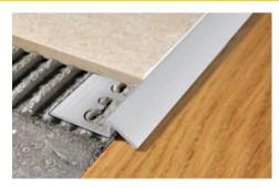
1. Choose the profile with the required finish. 2. Fill the profile cavity with adhesive and apply the adhesive onto the area of application.
