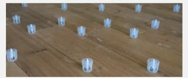
By turning the cap it is possible to level a thickness of up to 40 mm with an 8 mm joint.
