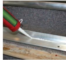
4 Apply adhesive as per manufacturer's instructions.
