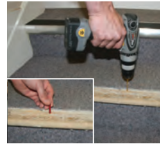
3 Drill and Plug to suit the screw size.
