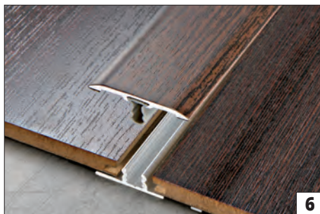
6) Place the profile over the "U" shaped channel.
