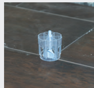
Linear leveler installation.
