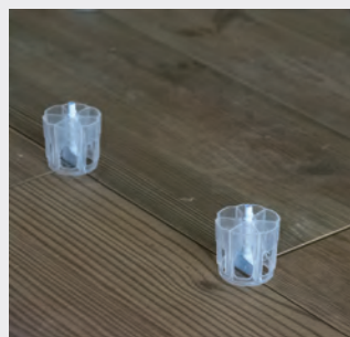
T-shaped leveler installation.
